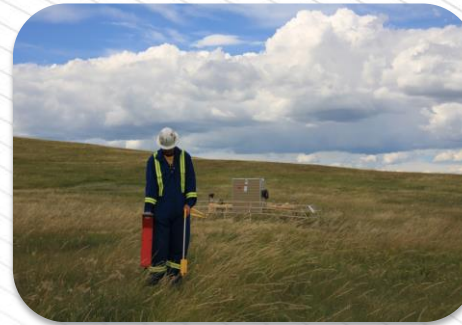
Buried Utility Locating
